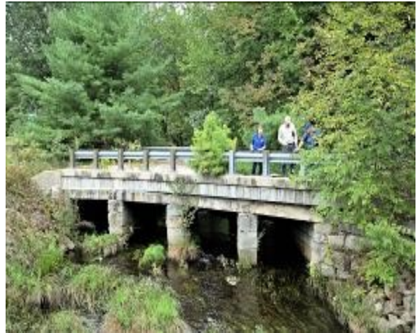
Assessing bridge clean-up September 2018. (Photo by Lion David McBee)
