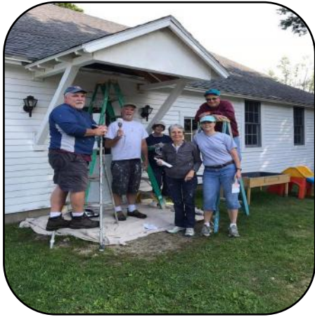
AB members restoring Grapevine Community Center
